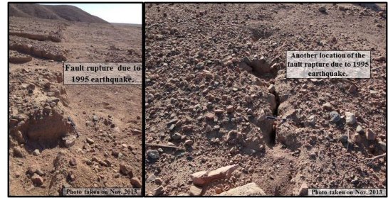
Figure 3: Two photos show the rupture due to the 1995 earthquake.
